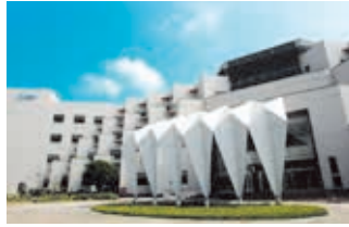
Tainan Plant (Diamond-rated Green Building)
